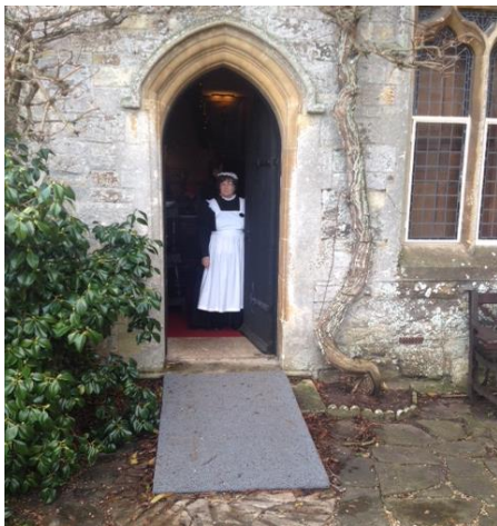
Fig. 21 – Private entrance to allow access to lower floor of Palace House.
