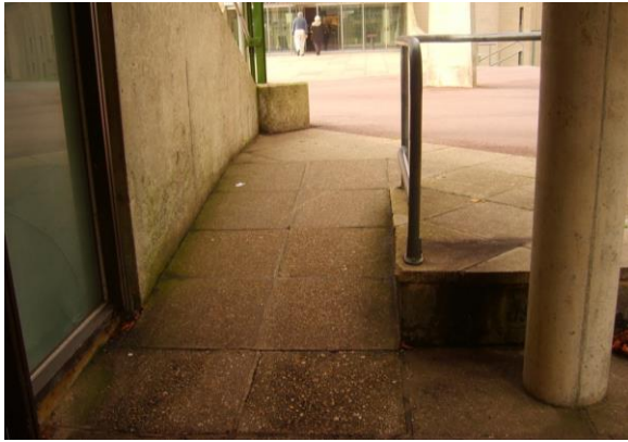
Fig. 7 – Entry to accessible lavatories from main pathway.
