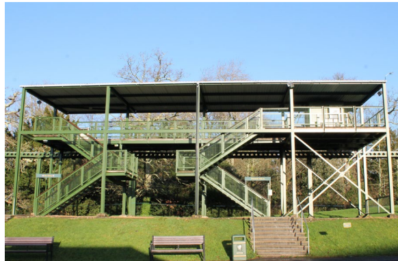
Fig. 26 – North Monorail Station
