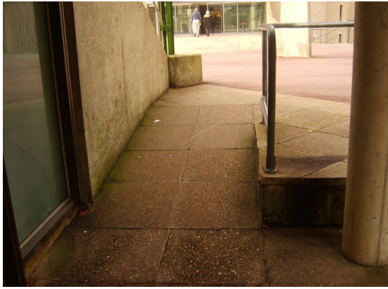
Fig. 7 – Entry to accessible lavatories from main pathway.
