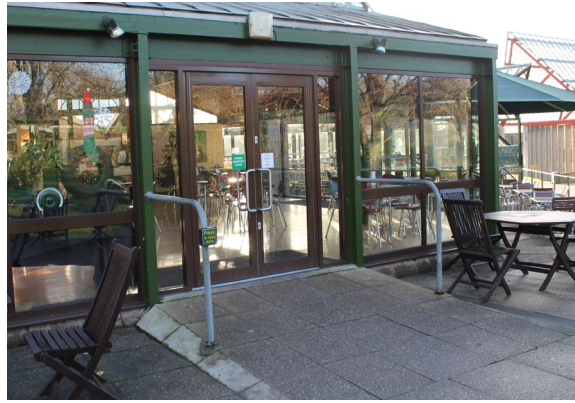
Fig. 8 – Power assisted doors to Brabazon restaurant.
