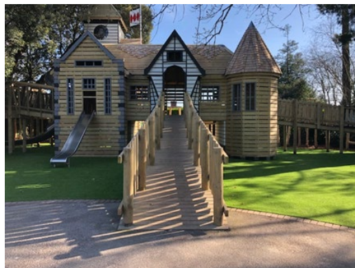
Fig. 28 – Ramp to Little Beaulieu main play structure
